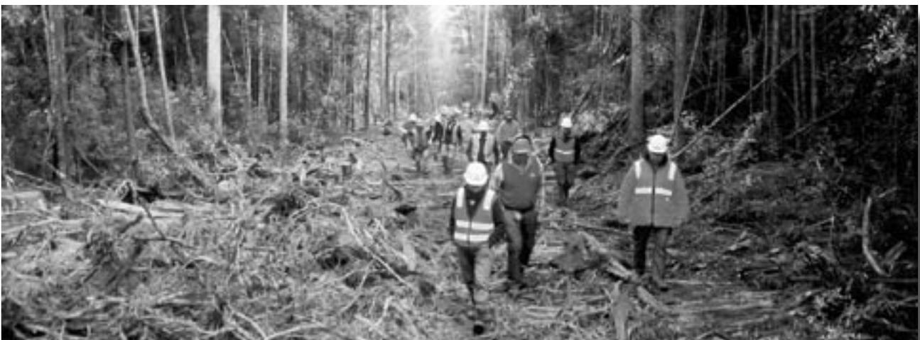
Figure 2. Primary snig tracks were cleared to a minimum width of about 9 m to allow an excavator to rotate at least 180 degrees. Slash was piled onto the cleared area to protect the soil and make a semi-permanent extraction path.
