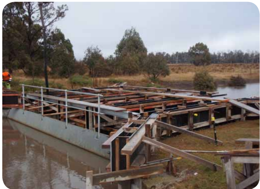
Figure 14. Lifting the height of the Lake Sorell screens
