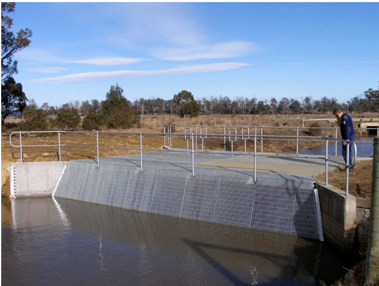
Picture five: Completed Lake Sorell outlet screen duplication. This structure ensures all water released from Lake Sorell in passed through mesh screens to prevent carp being transferred between lakes.
